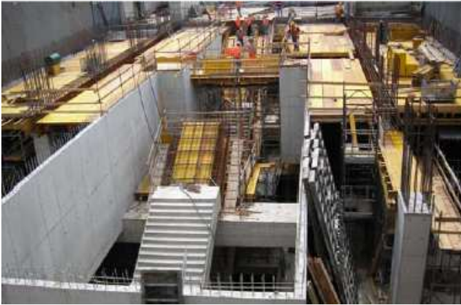
Brescia Metro: Typical Station Construction
