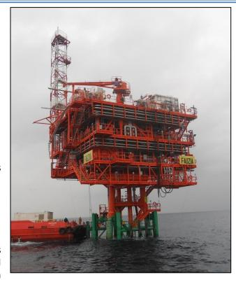
The Fauzia platform is provided with two 30" double completion wells and one conductor spare. A 12" export riser connects the platform to existing Barbara B platform. The total weight is 675 t.
