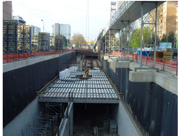
Line 5 BIGNAMI station – mezzanine deck
