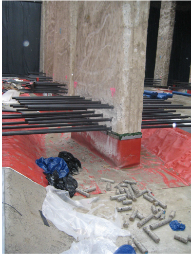
Line 5 Slurry concrete diaphragm connecting rebars to deck
