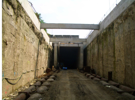
LINE 2 Concrete caisson gallery – pushing from back with jacks
