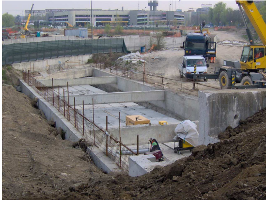
LINE 2 Concrete caisson gallery 70m long pushed under highway
