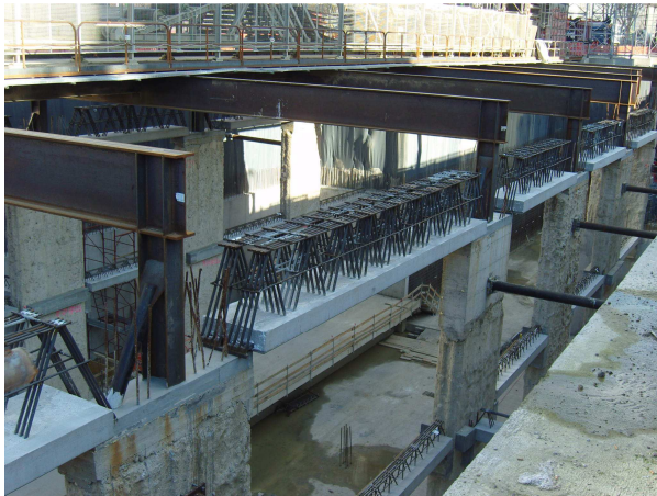
Line 5 Prefabricated steel/concrete beams "REP" system
