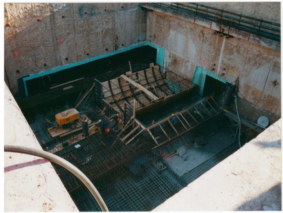
Line 1 FIORENZA well – TBM starts slab
