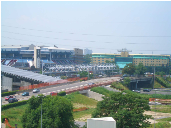
LINE 2 Pedestrian bridge over the highway Overall view
