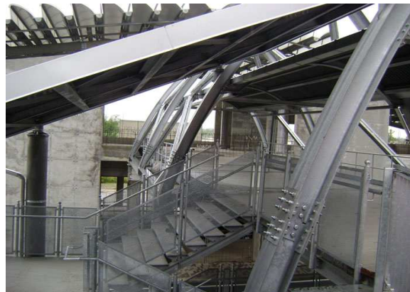
LINE 2 Pedestrian bridge over the highway Details
