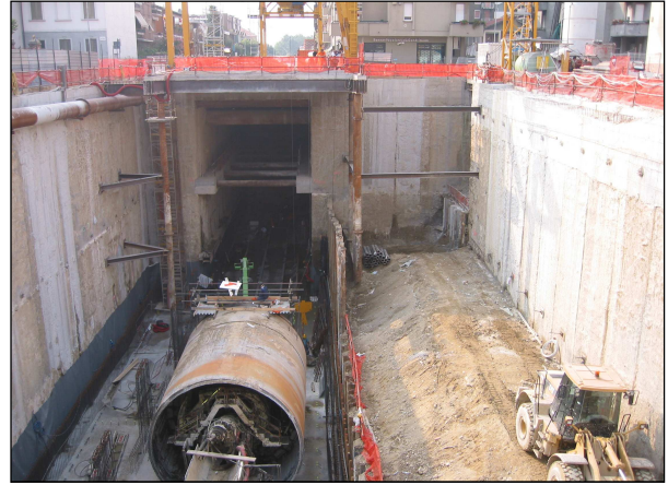
Line 1 TBM passing in PERO station
