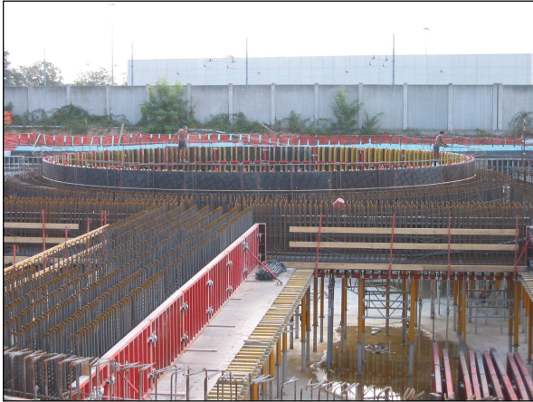
Line 1 – Station of RHO Large architectural roof opening
